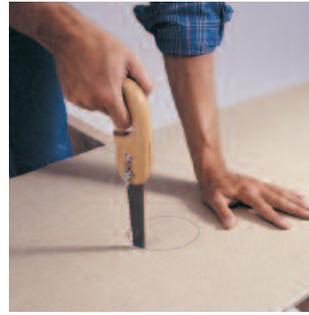
**Curved Cuts** can be made easily with a keyhole saw. If an area must be cut from the center of the board, it is recommended that a hole be bored that will take the point of the saw.
