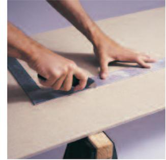
**1. Cut Decorative Surface** with a sharp knife to a dimension of 1" wider than the panel width desired. Then turn vinyl surface face down.
