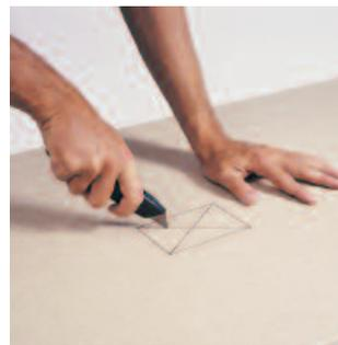
**Electrical Outlet Box** openings can be made easily by cutting the Durasan as shown by the solid lines in the picture above. Strike a sharp hammer blow to the "X". Cut away back paper.
