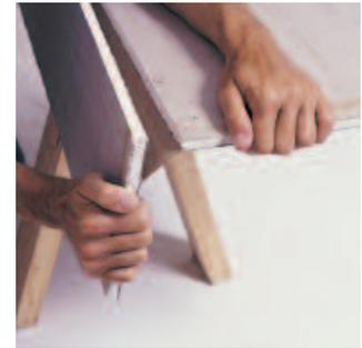
**2. Score Back Surface** with knife to the desired panel width. Snap gypsum core and peel this 1" piece from decorative surface. Smooth core if uneven.
