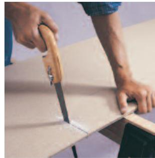
**Where Two Cuts Join**, one cut must be made with a saw, the other cut can be made by scoring and snapping. Cuts like this are required around door and window openings.
