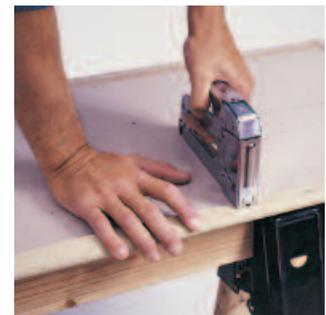
**3. Wrap** the excess flap of vinyl over the exposed gypsum core and staple to back.
