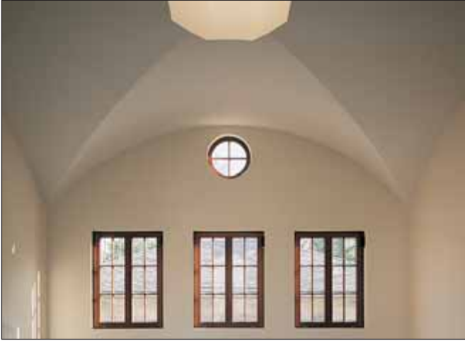
Veneer plaster expands architectural design limits as with this curved vaulted ceiling.
