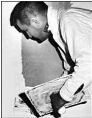
Kal-Kote is applied in 2 coats, a base and a finish, to form a hard-surfaced, 1/8" total thickness.
