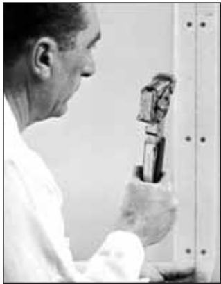
Joints are reinforced with Kal-Mesh fiberglass webbing. Steel corner and casing beads protect corners.
